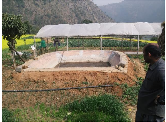
Soil Cement Tanks
