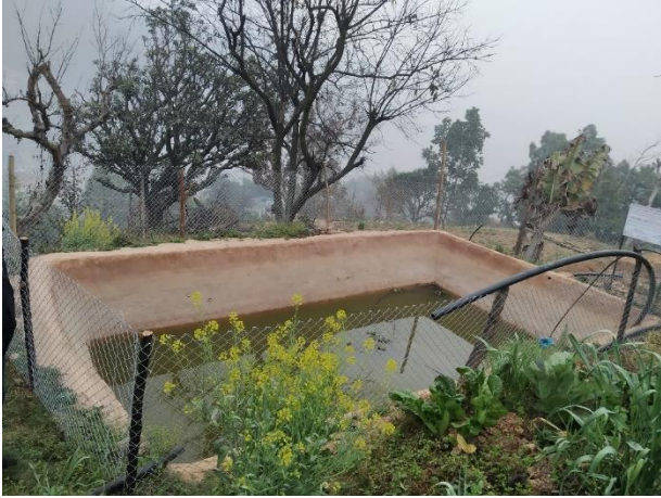
Soil Cement Tanks
