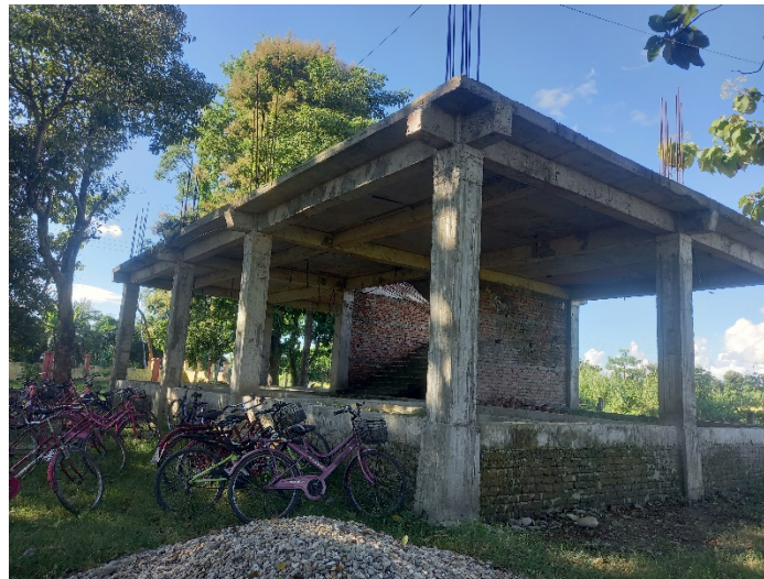
Figure 48: Ongoing construction of flood resilience school building
