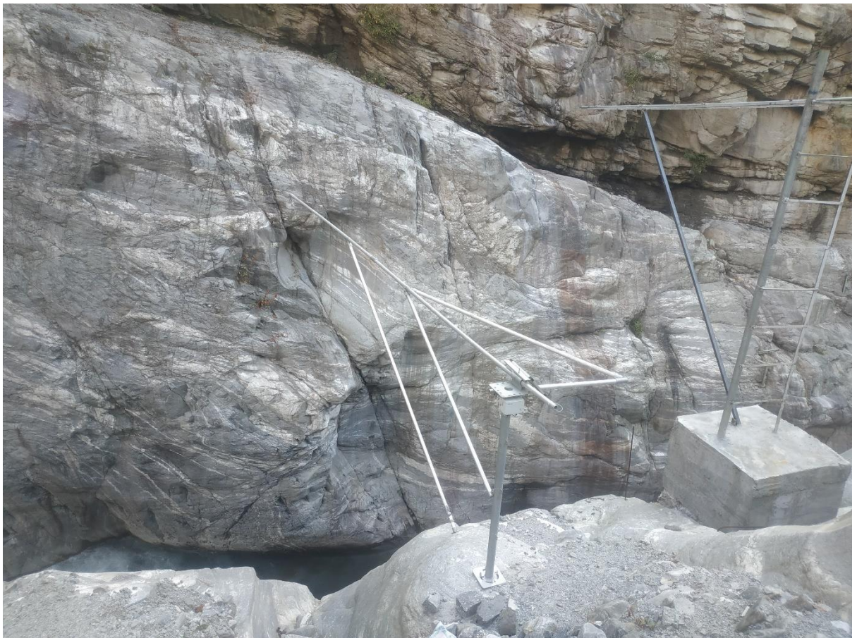
Figures: Automatic weather station and River level sensor in the upstream of melamchi
