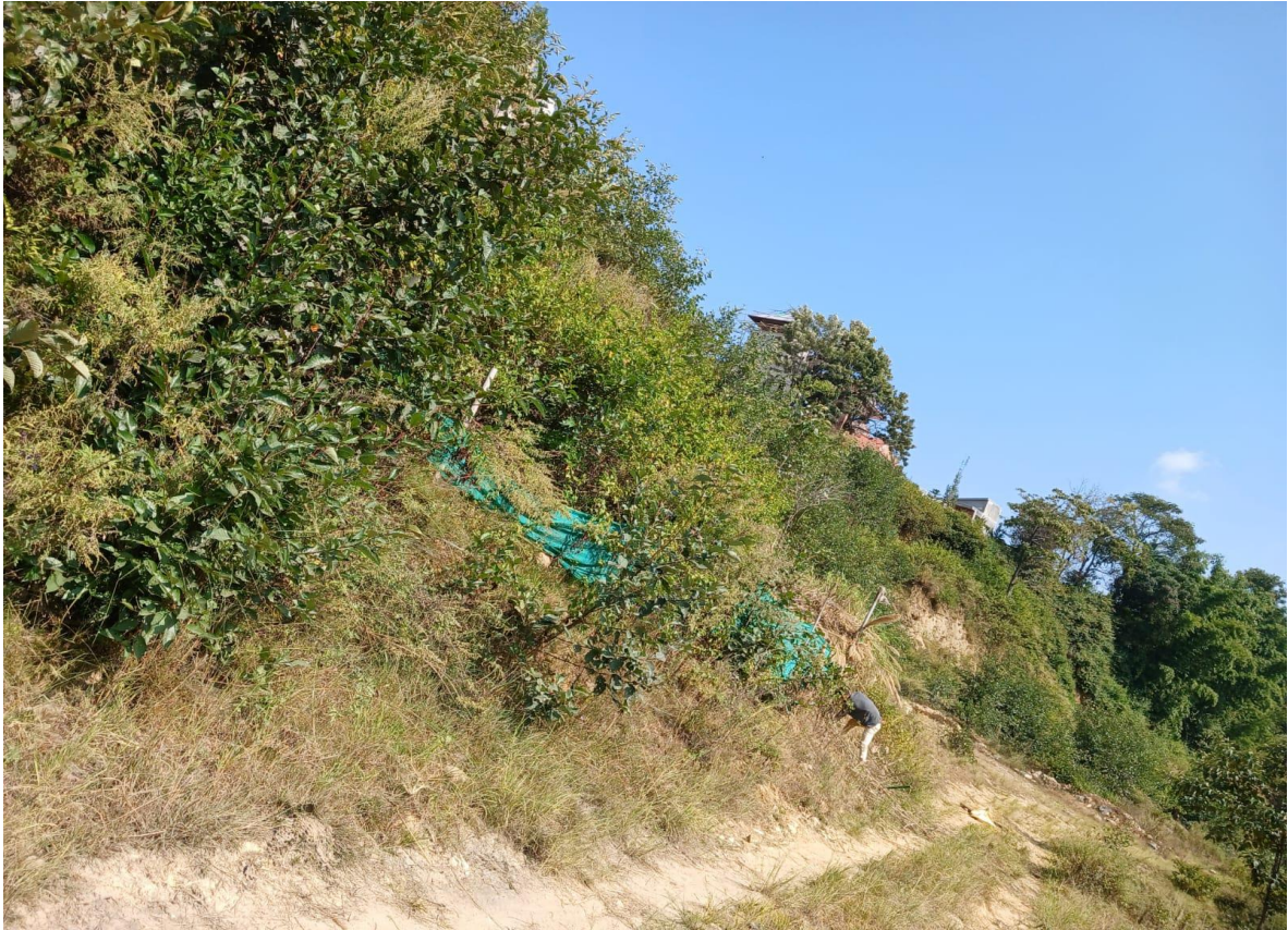
Figure 3-9: Firfire Danda Landslide Image
