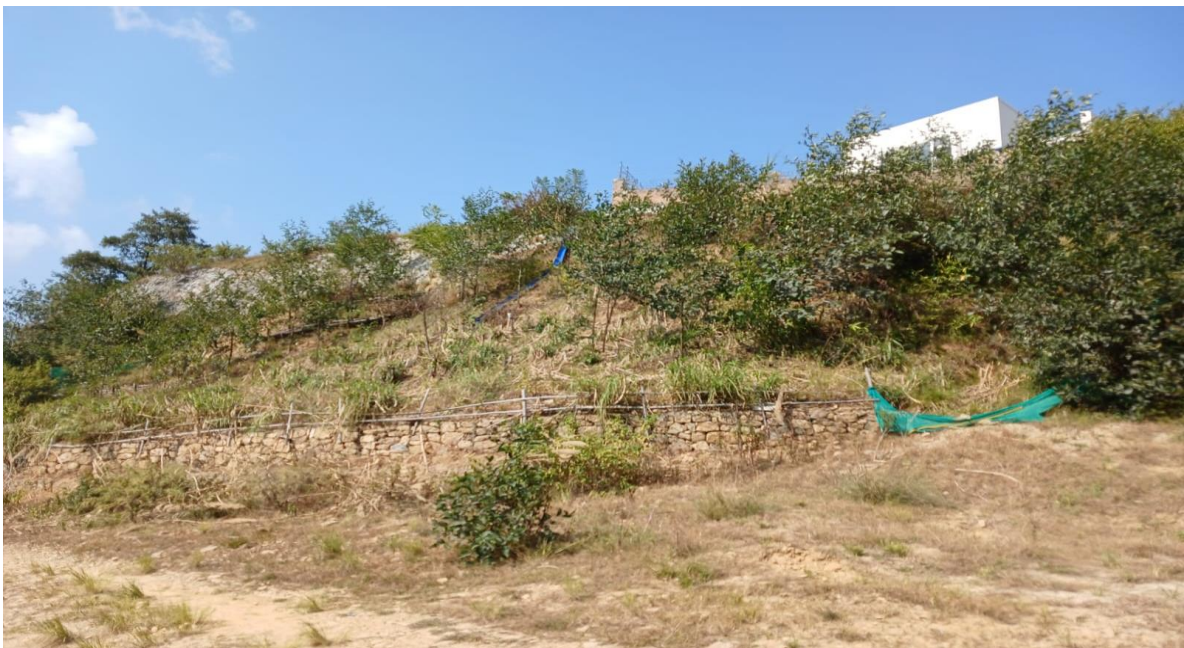
Figure 3-6: Soil Profiles in Firfire Dada Landslide area after the plantation.
