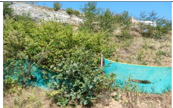
Photo Plate-2: : Firfire dada Landslide Site photo
