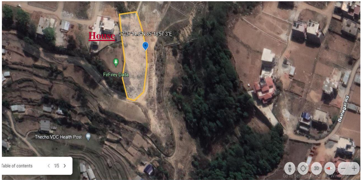
Figure 3-2: Google Photograph of the study area (note the house under the threat of slope failure)
